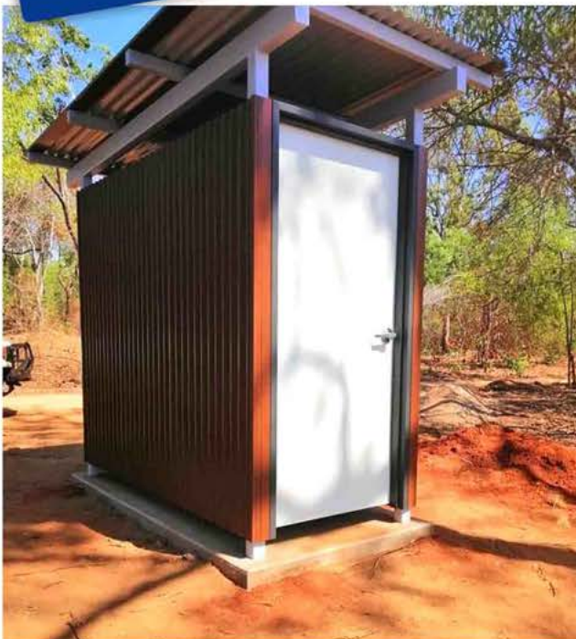
First job done - Installed toilet facility
